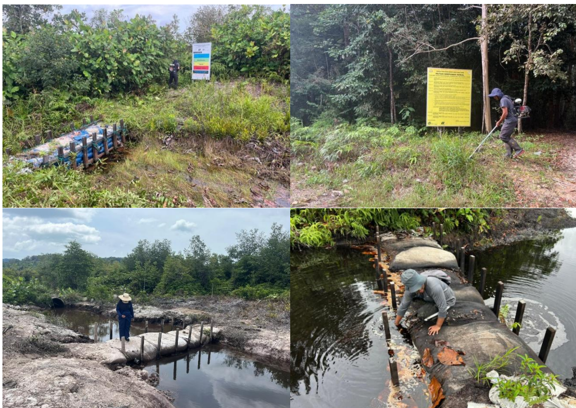
Figure 8. Maintenance of conservation signages and monitoring of the check dam structures were carried out to ensure that all installations remained in good condition and continued to function effectively. Regular inspections helped verify the structural integrity of the check dams, enabling them to retain water efficiently, maintain peatland moisture, and support hydrological restoration within GAFFR.
